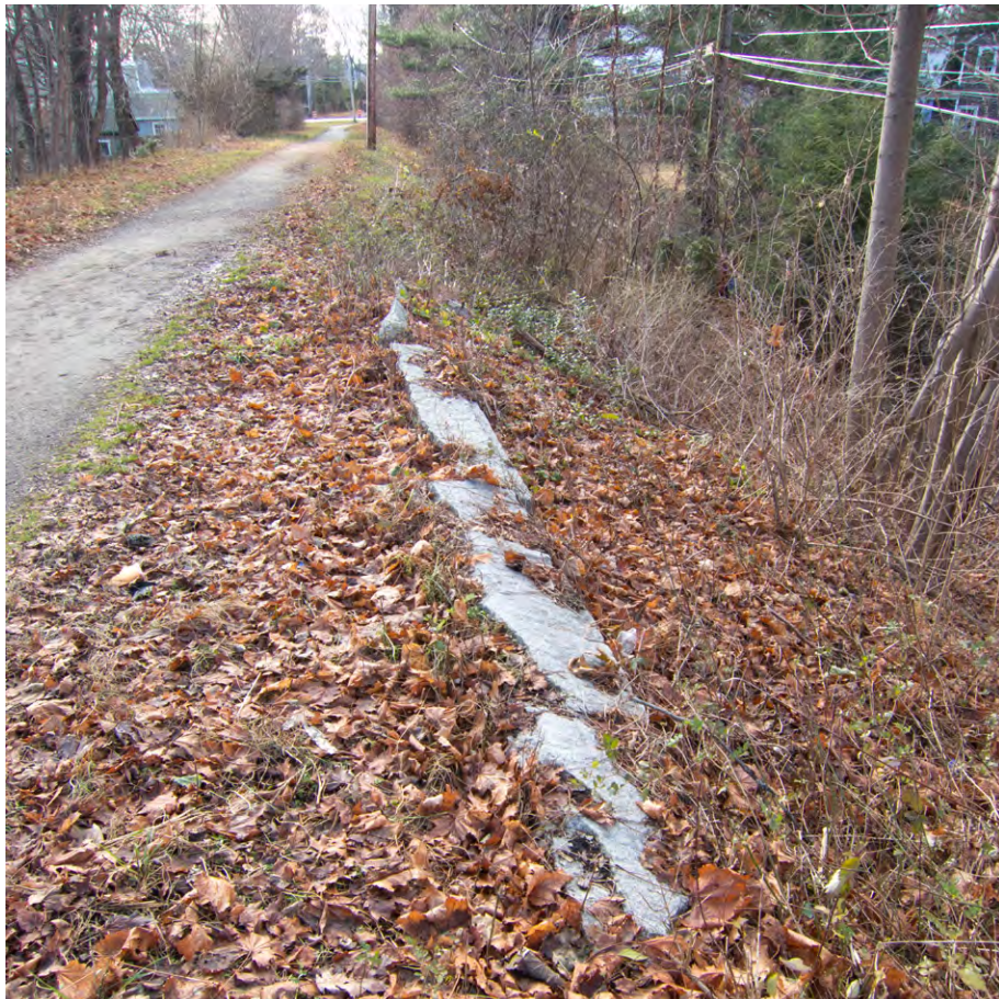
Curbing along The Path between Pleasant and Maverick Streets was put in for erosion control.
