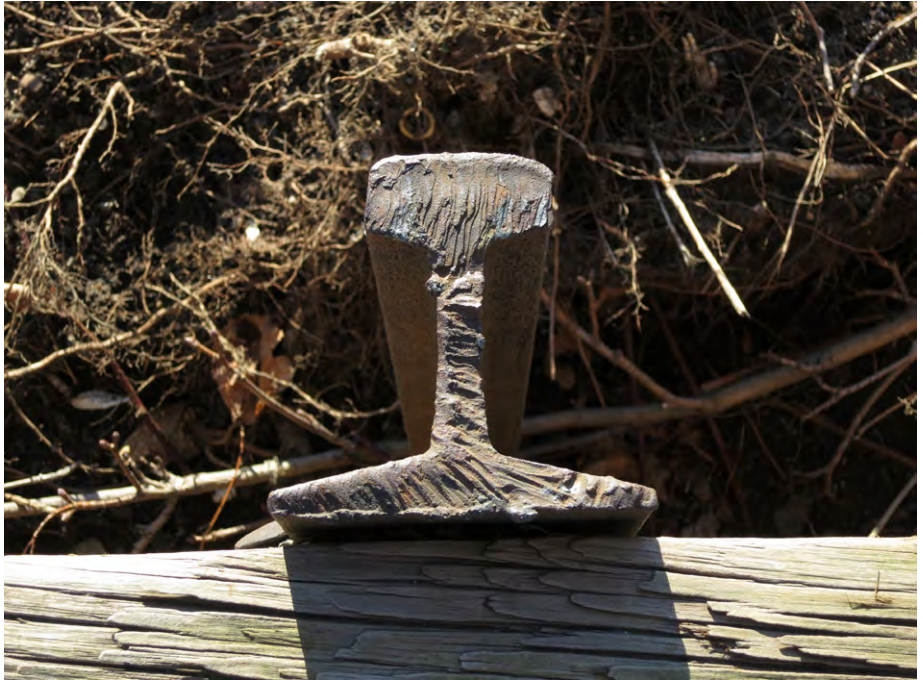
One of the many old rails reused as fence posts along Roundhouse road.
