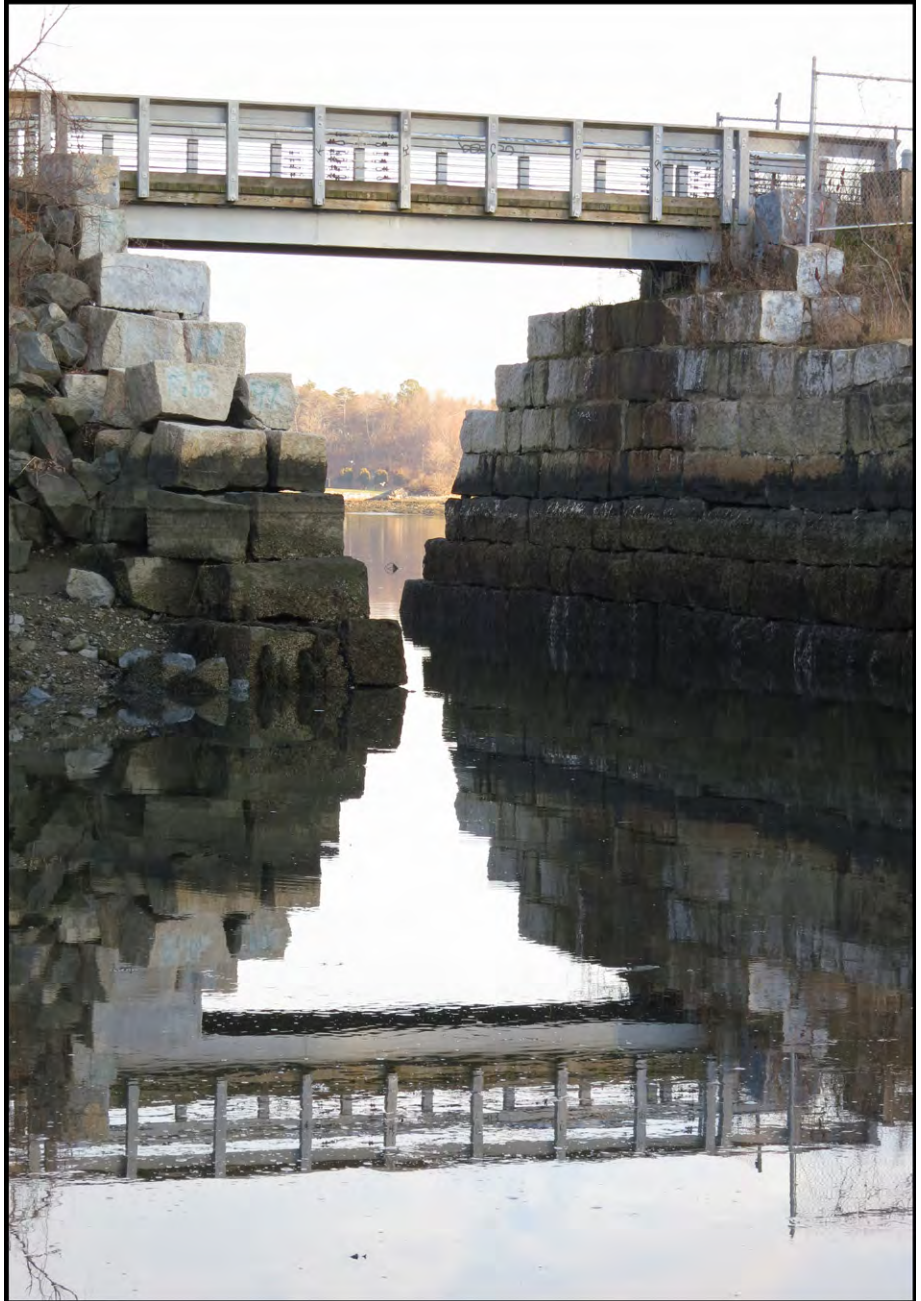
The original bridge over the Forest River at Lead Mills is long gone but a pedestrian bridge now crosses the Forest River using the original foundation. The two pedestrian bridges in this area were built because a new power line from Salem had to be buried. To "bury" the cable in these two open areas the bridges were built with the power cable running underneath them.
