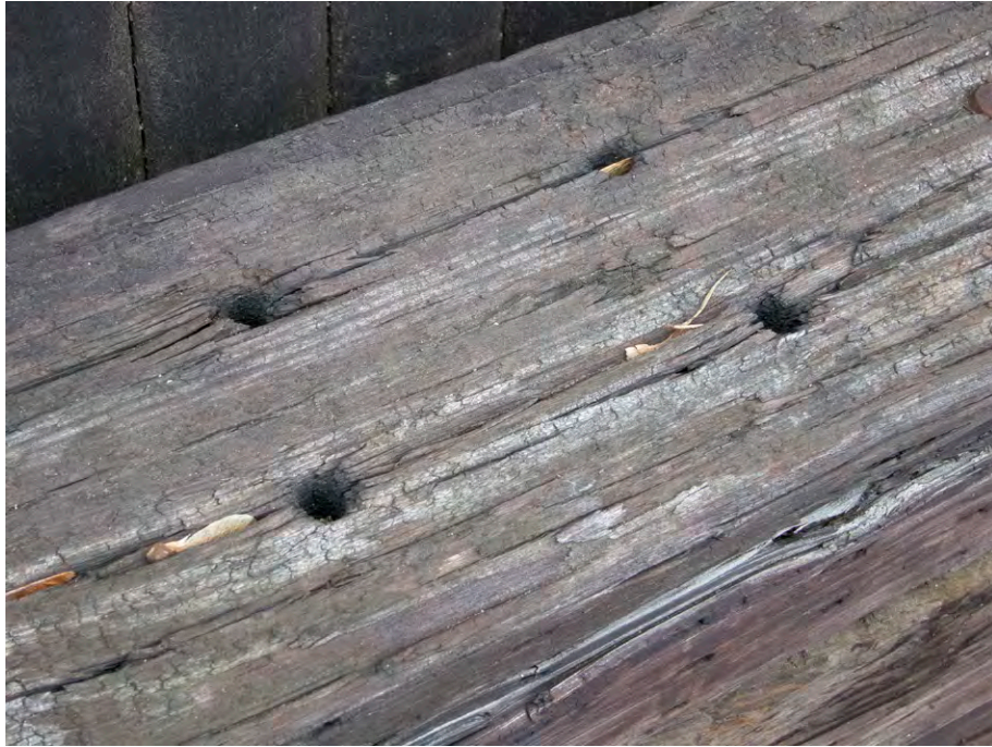
Along Roundhouse Road you will find retaining walls made using recycled railroad ties with the signature four-hole pattern where rails were attached with spikes.
