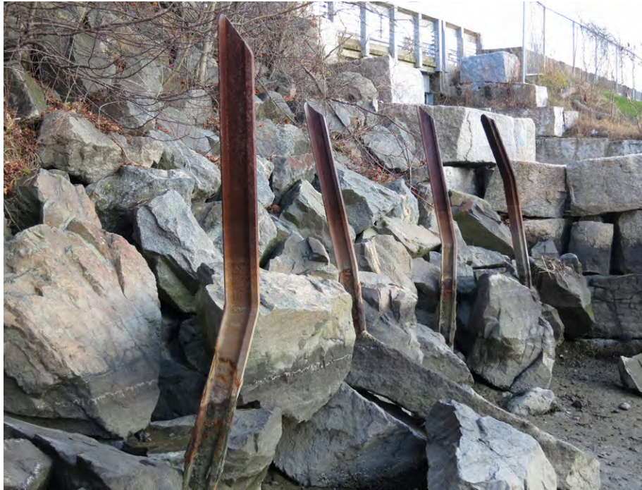
Rails have been used to hold riprap in place below the bridge.
