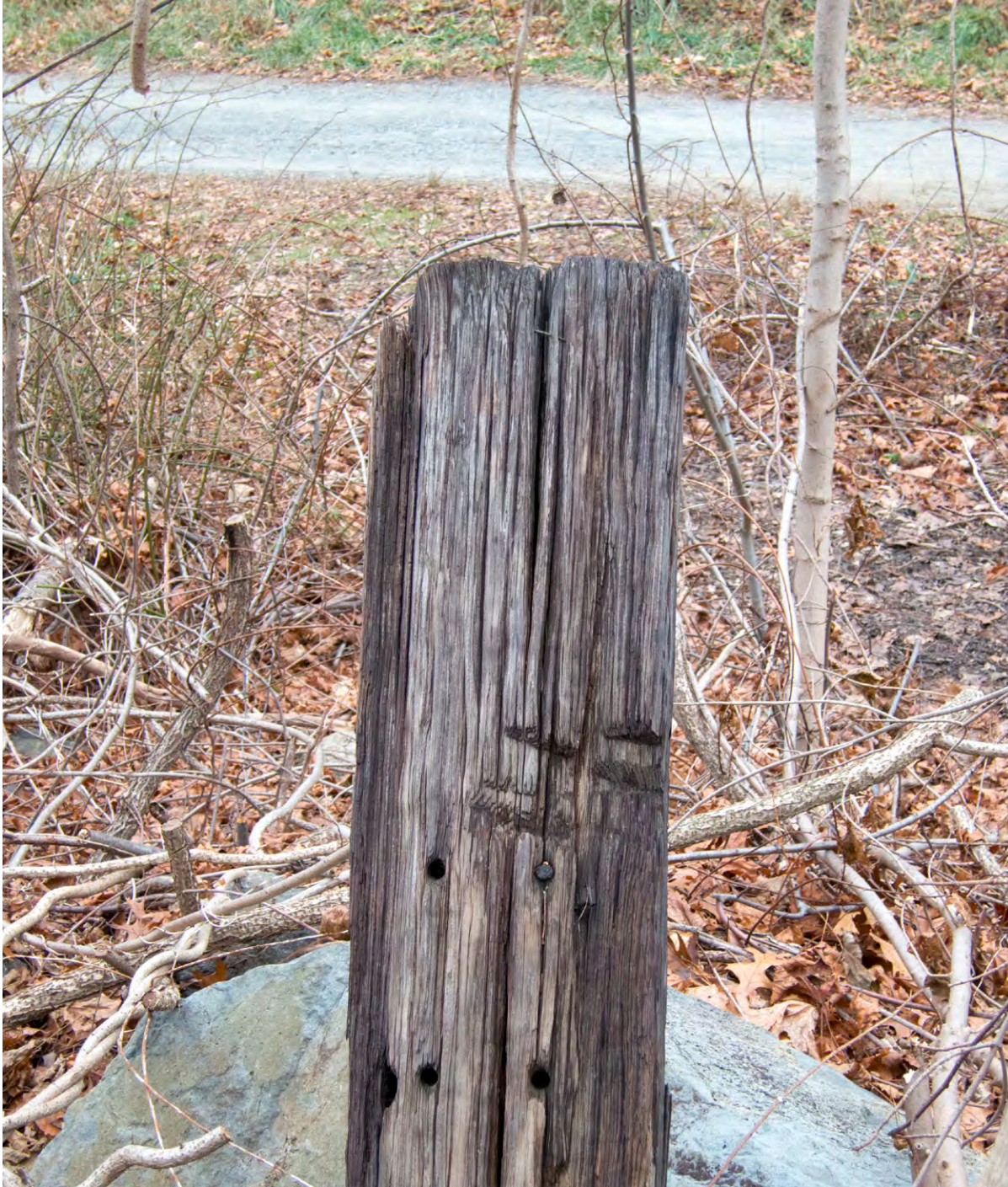
This tie is upright at the intersection of the Salem Branch and the cut through at Wye Pond. You can see the four hole pattern where a tie plate was attached and The Path can be seen in the background.
