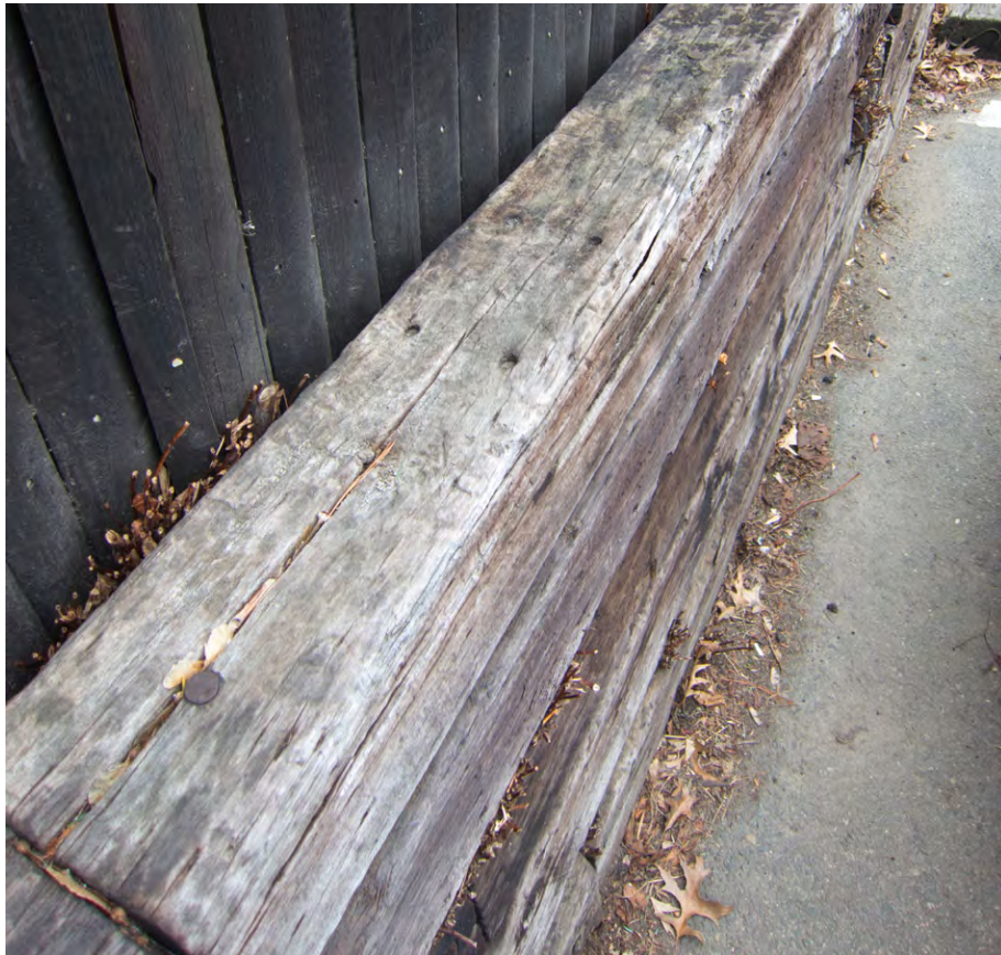
Ties reused as retaining walls along part of the road.
