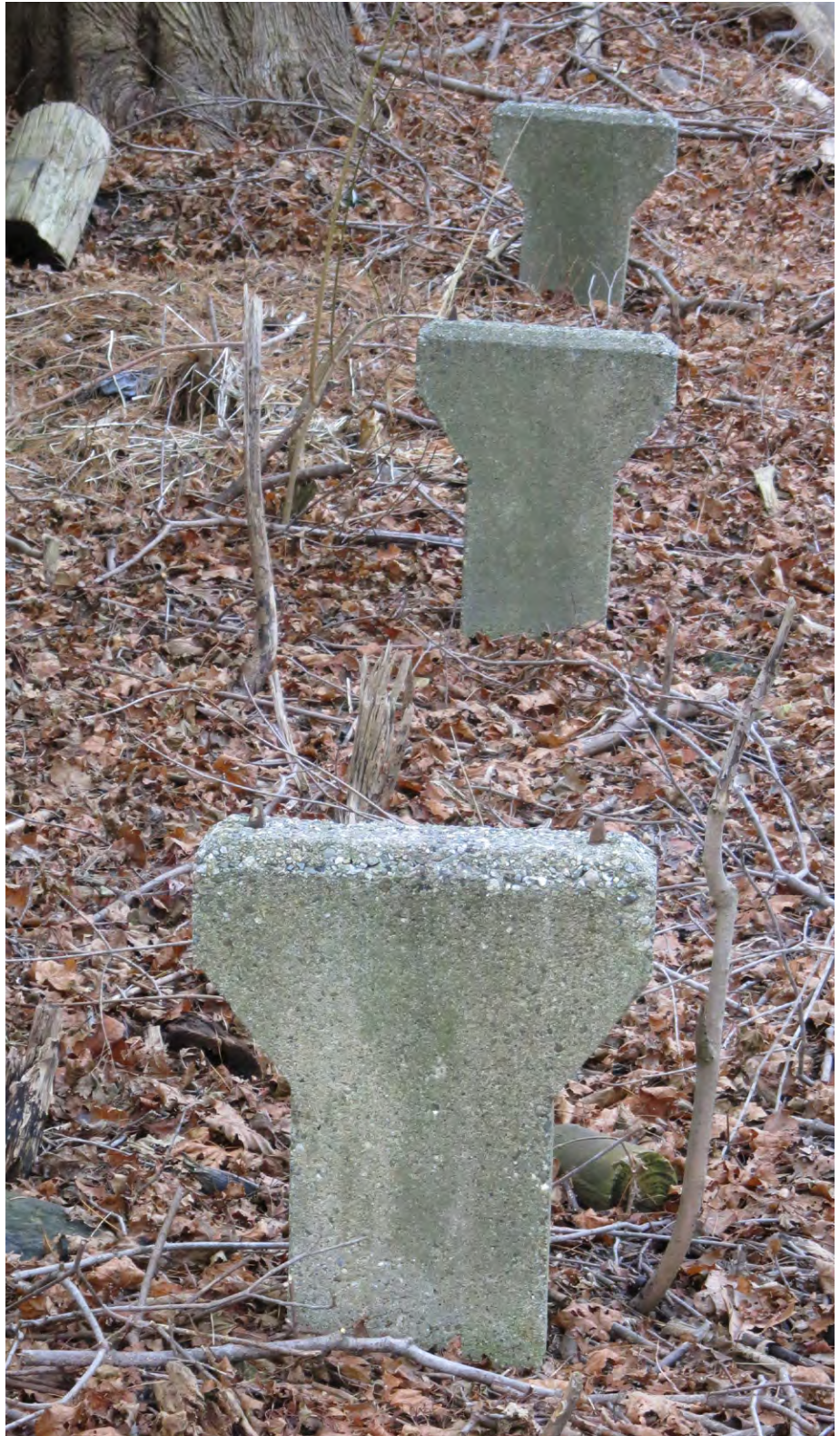
These three stands at the end of Briar Lane once held spare rails in case any needed to be replaced.
