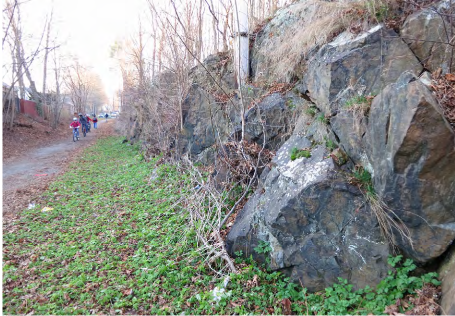
A rock cut between Pleasant Street and Smith Street. All along The Path you will find cuts such as this as well as raised portions—all needed to keep the rail bed itself as level as possible.
